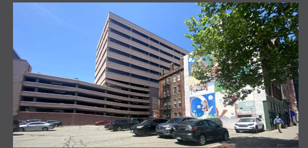
Attached parking garage located behind the building.
